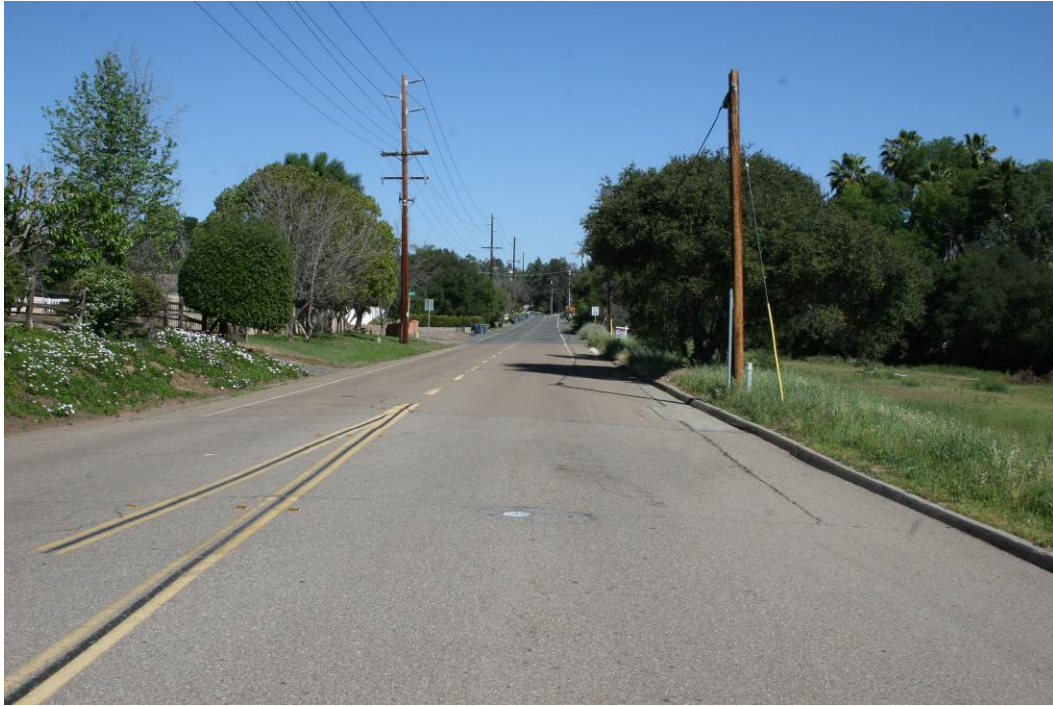
Photograph 17: Existing view looking north along Encino Drive (at approximate MP 27).
