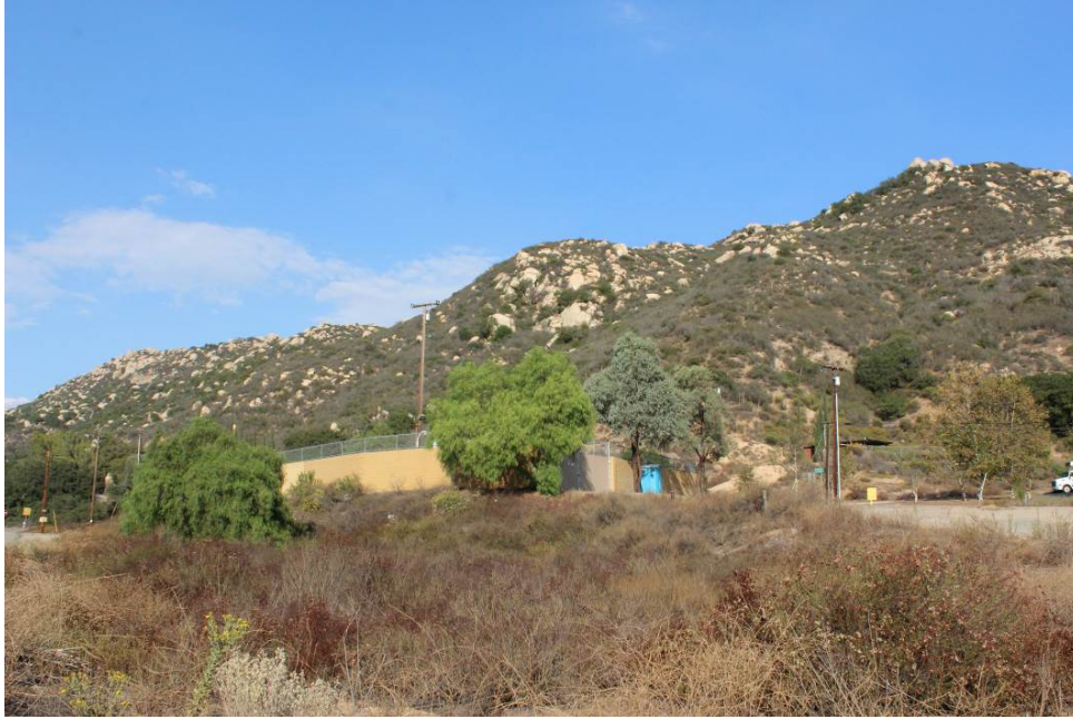
Photograph 1: Rainbow Metering Station and location of the proposed Rainbow Pressure-Limiting Station (northern terminus of the Proposed Project), looking northeast from Old Highway 395.
