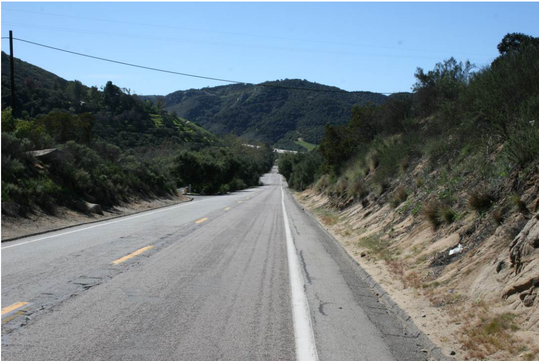
Photograph 10: Existing view looking southwest along Old Highway 395 (at approximate MP 12.1)
