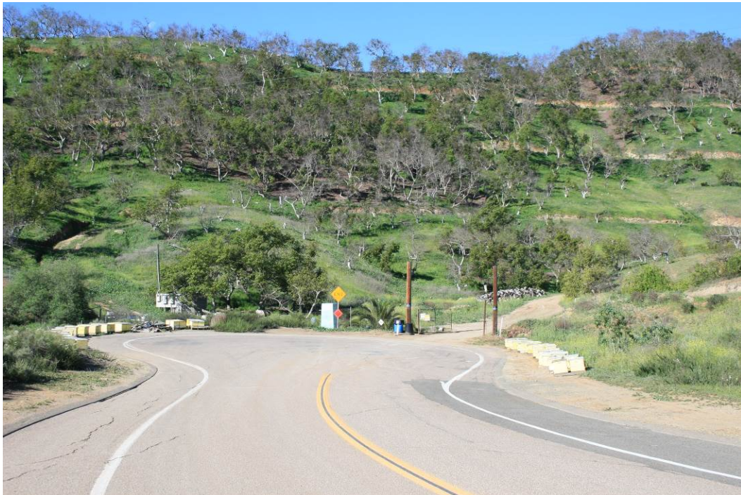
Photograph 4: View from the southwestern end of Rainbow Hills Road looking southwest, where Laydown #2 will be located and where cross-country installation of the Proposed Project will occur (at approximate MP 3.3).
