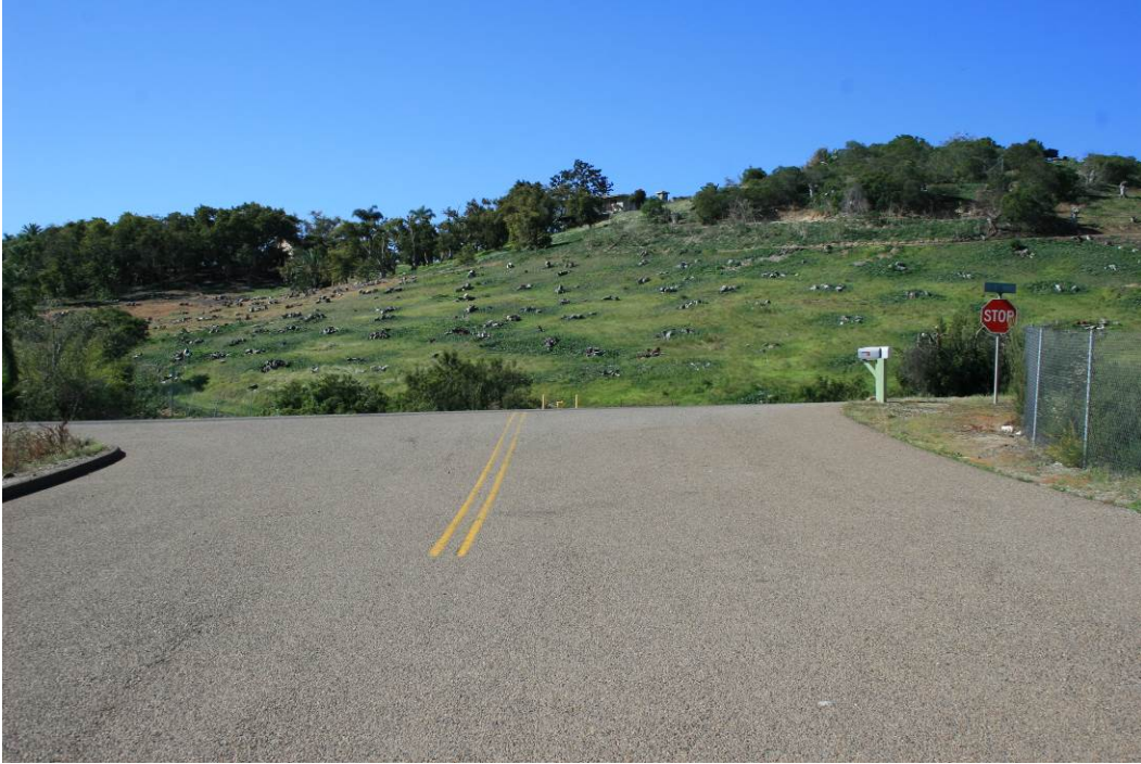
Photograph 5: View from approximate MP 3.8 facing south toward Mission Road (a San Diego County-designated scenic roadway).
