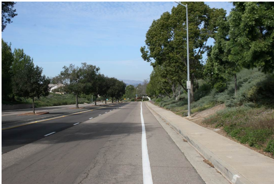
Photograph 19: Existing view facing north along Pomerado Road (at approximate MP 31).
