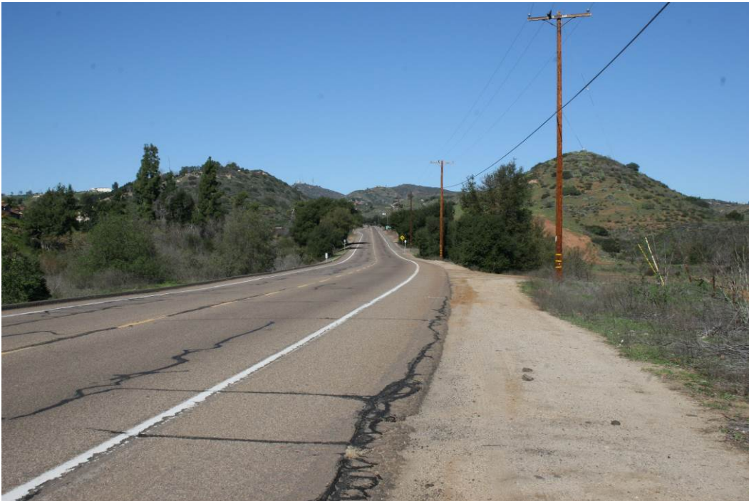
Photograph 6: The location of proposed MLV 2, looking north-northwest along Old Highway 395 (at approximate MP 6.2).
