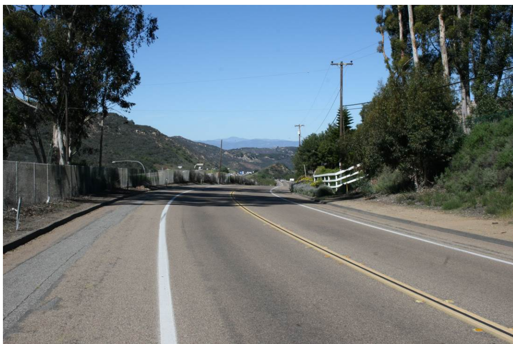
Photograph 12: Existing view looking northwest along Old Highway 395 (at approximate MP 18).
